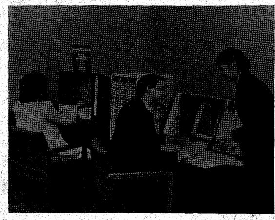
which cartridge in the Magazine Collection contains the full text of the material and the frame number on which the article begins. The user simply selects the appropriate cartridge from the Magazine Collection carousel and snaps it into the system's viewer/printer. The user presses a button to advance the film to the appropriate frame number, then he or she can read the article on the viewing screen or press another button to print a permanent copy of the material
