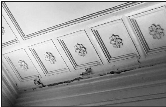
Repair of the damage to gallery spaces on the third floor and in the library stacks has now been completed.
