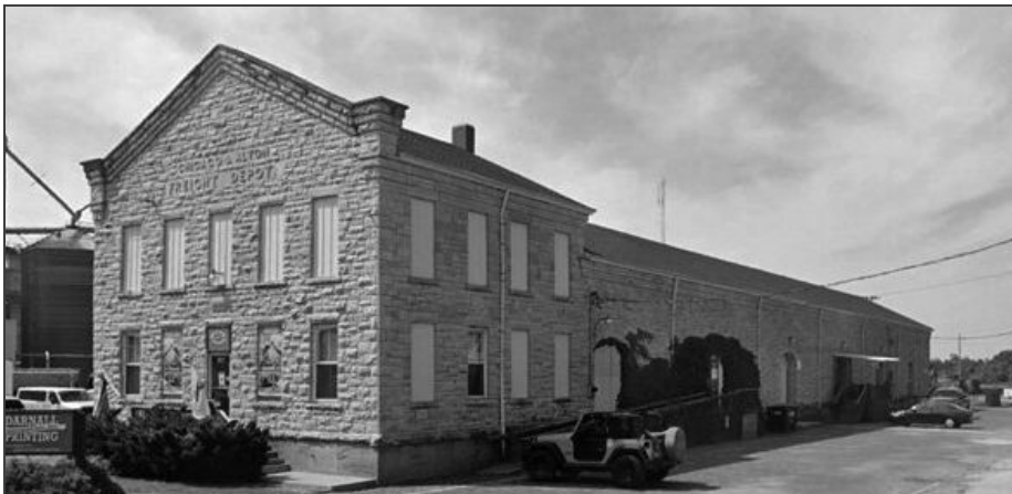
The Chicago & Alton Railroad Freight House, located at 801 W. Chestnut St., was completed in 1888.
