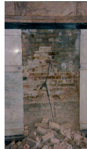
Creation of a doorway between the library stacks and the reading room.
